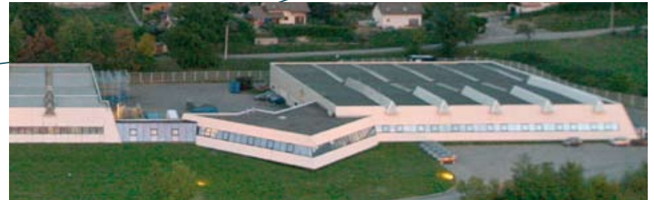
Aix-les-bains head office
